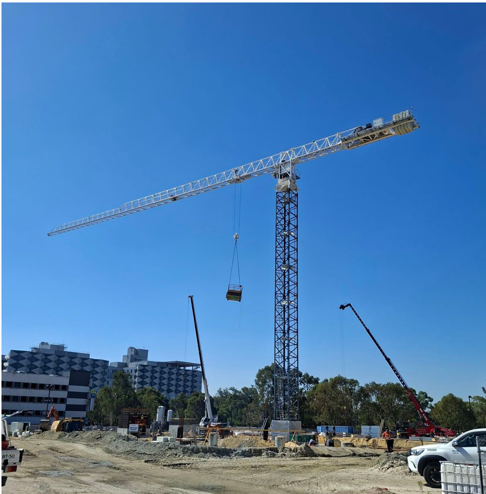
Crane in operation at the new car park
